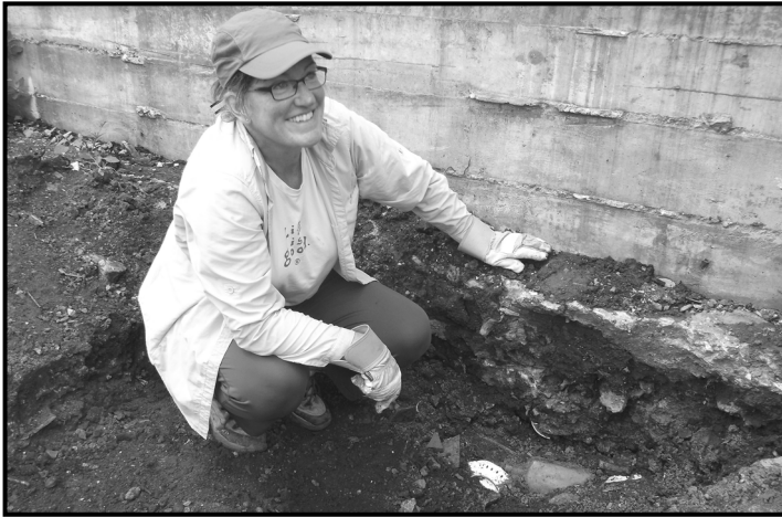
MHAHS Curator and (fortuitously!) trained Archaeologist Johnna Buysse excavates and documents a privy site unearthed during construction of the Driftless Historium history campus on the 100 block of Mount Horeb's Second Street.
