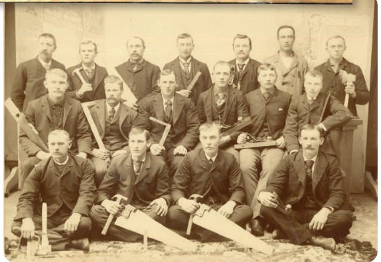
Kleven Brothers construction crew, c. 1890. Knut is in the middle of the back row, and his brother Gilbert is third from the left in the second row.
